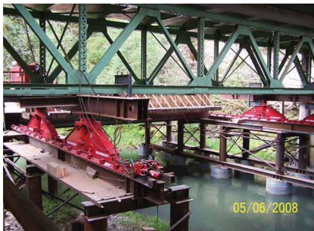
View of a complete hydraulic sliding system
