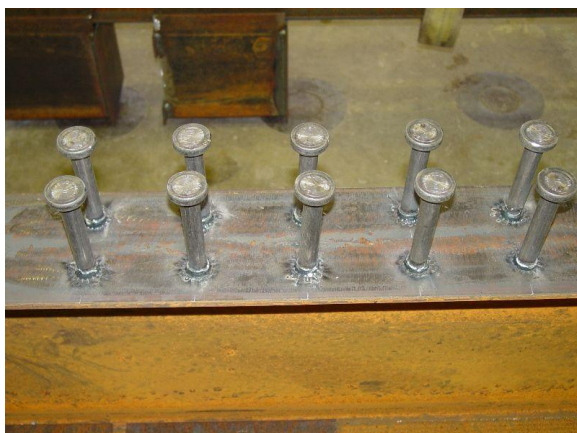
Shear studs
