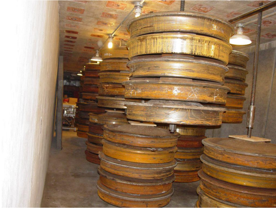
Figure 3-34. Stacks of ballast loads in the basement.
