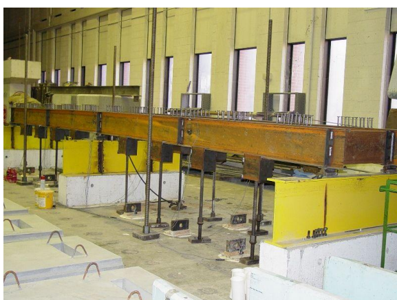
Overview of displaced girder
