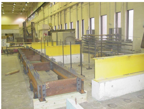
Girder ready to placement
