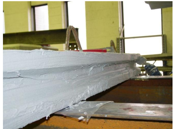
Epoxy matching cast shear key
