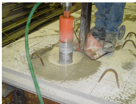
4" diameter core driller
