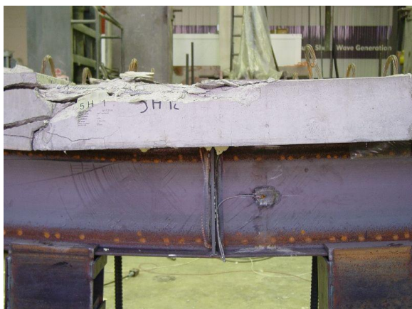
Precast panel (west mid-span)
