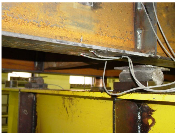
Shim removal (begin)
