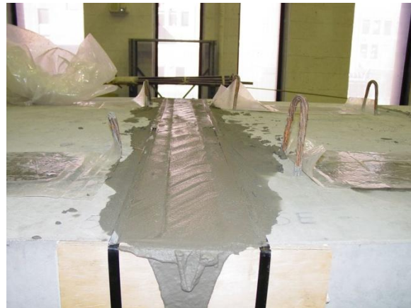
Grouting closure region
