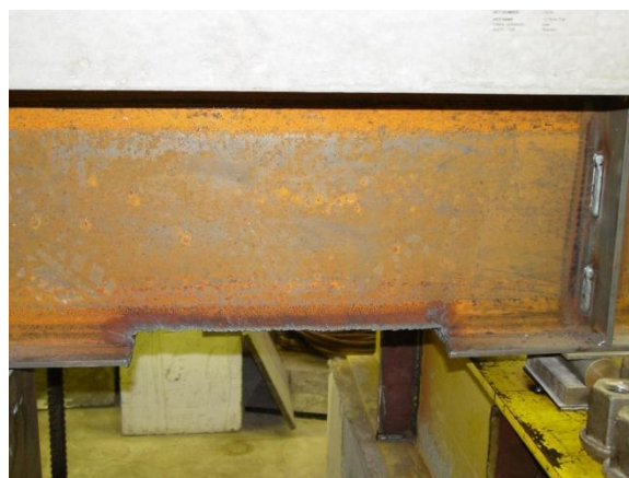
Bottom flange after the cut
