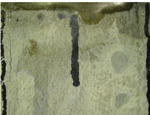
Close-up at closure region
