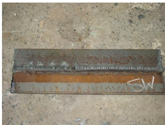
Torch cutting the bottom flange
