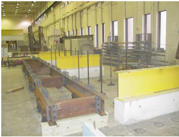
Assemble of girders and bracing system
