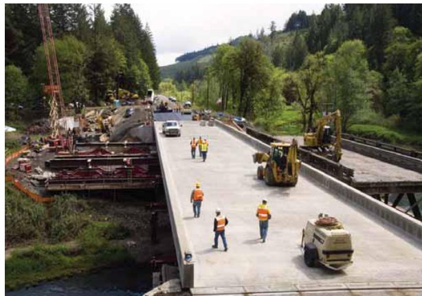
Replacement of superstructure and end panels.
