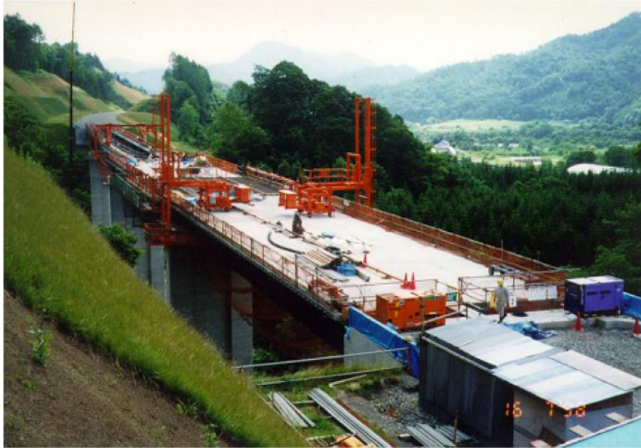
Figure 2-6. Concrete Casting with Movable Form at Chidorinosawagawa Bridge (Nagai, et al., 2000).
