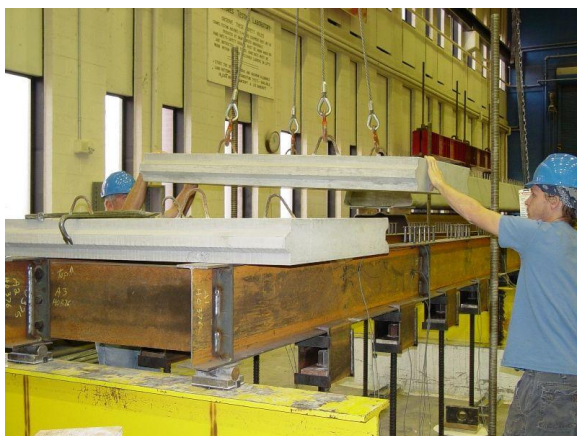
Placing 2nd panel
