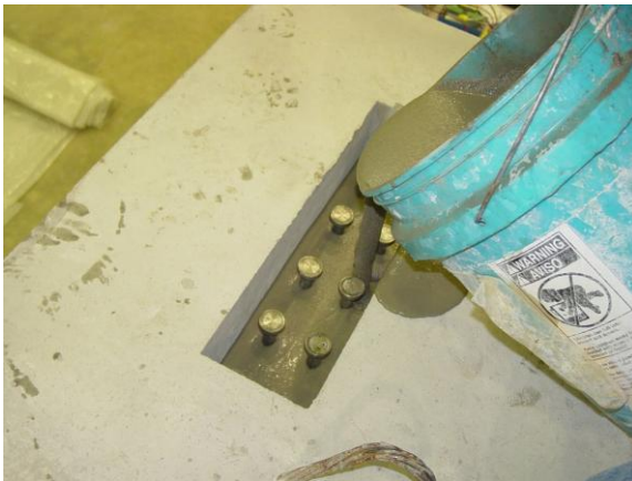
Grouting shear studs blockout
