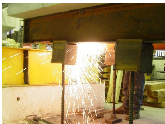
Torch cutting the bottom flange
