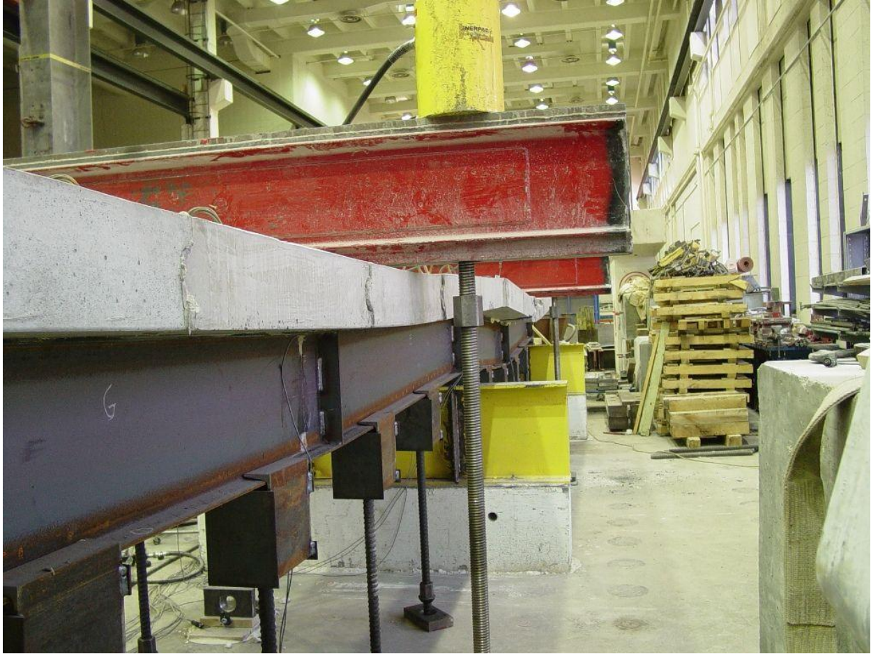
Figure 4-32. Large deformation due to yielding of bottom flange at mid-span
