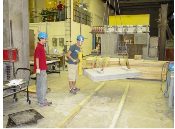
Precast panel being placed on sequence
