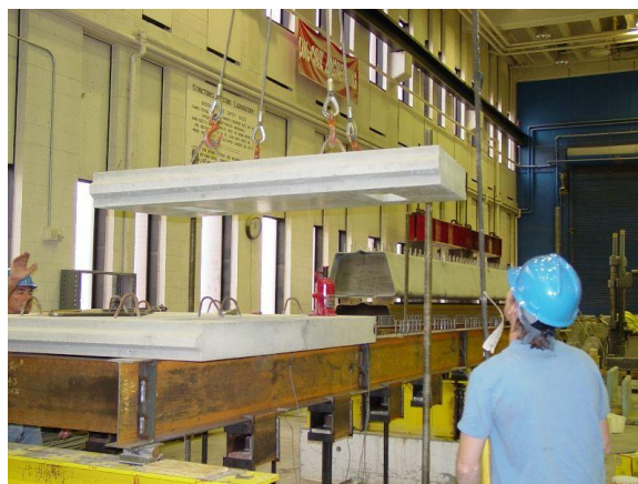
Placing 3rd panel
