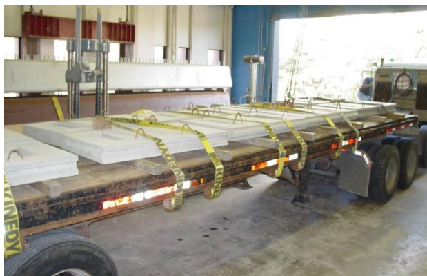
Precast panel delivering
