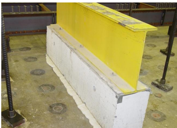
Supporting beam leveled with hydro-stone
