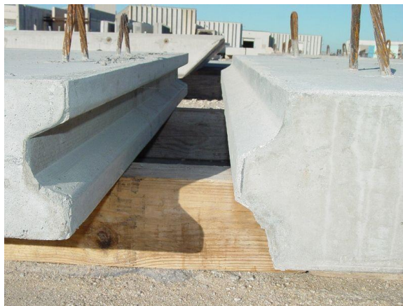
Shear key detail
