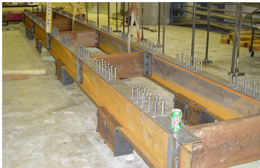
Final assembling of girders and bracing system.
