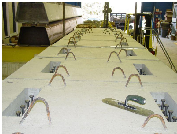
Top of the panel
