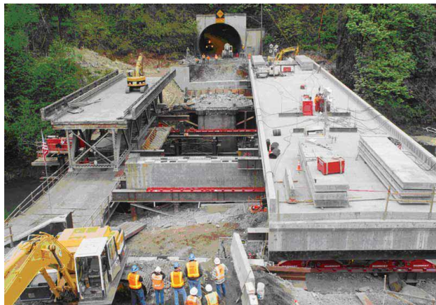
View of old and new superstructures
