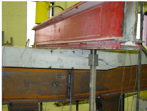
Concrete crush at west mid-span (north)
