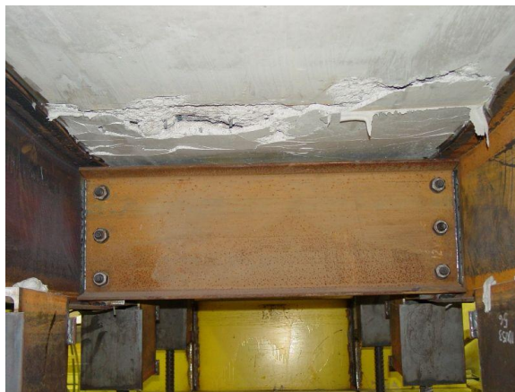
Precast panel (underneath)
