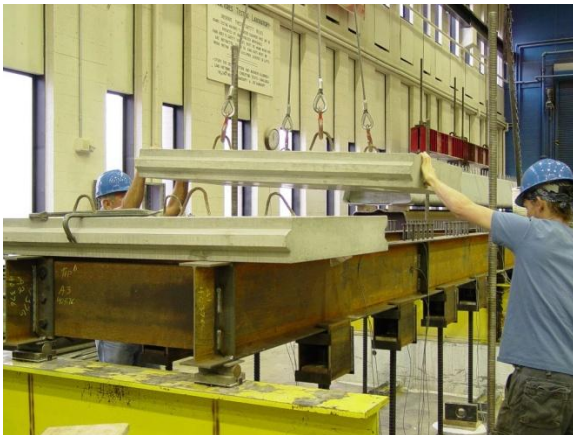
Placing precast panels
