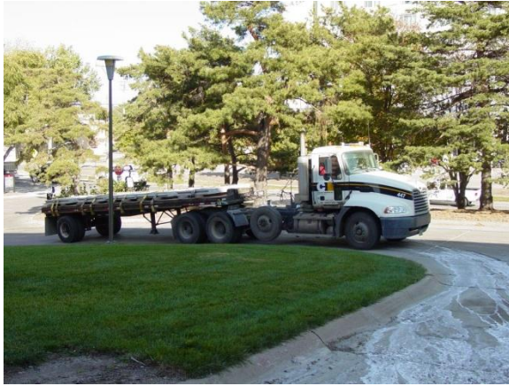
Delivery of 10 precast panels
