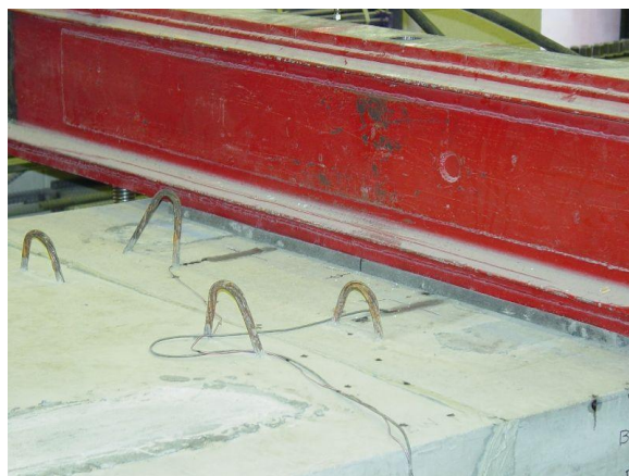
West mid-span (top view)
