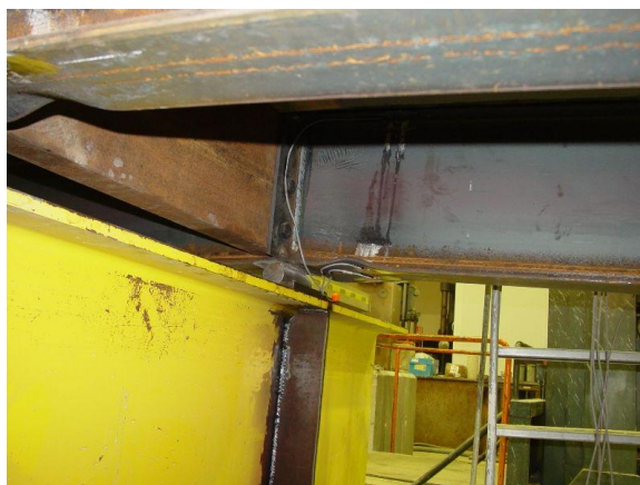
Interior support (underneath)
