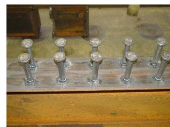
Shear studs
