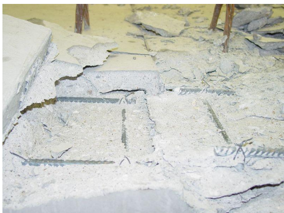
Precast panel reinforcement
