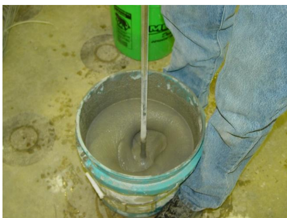
Mixing grout using power drill
