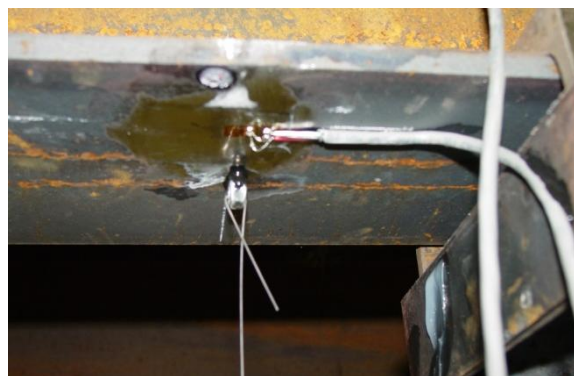
b) String line from the bottom of girder
